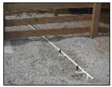
With the sprinkler heads temporarily installed, test the system before burying the pipes and installing the mats.
