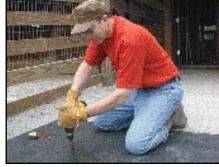
Rubber mats provide mud-free, slip-resistant footing. Drill holes for the pipes to come through, then install the sprinkler heads permanently.
