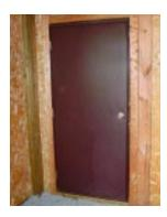
Exterior access doors should be insulated and have very good weather seals.
