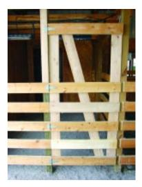
To begin the process of installing a climate controlled stall, first install the posts for doors and the wall supports. Next, attach the board fencing and all doors.
