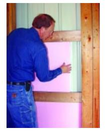
To insulate the exterior walls, you can install solid foam insulation. The top and bottom foam panels are in place. The center foam panel will be added next.
