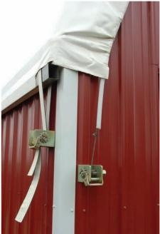
Above: The fabric is stretched tight over the top and down the sides of the buildings and also kept under tension by a system of cables, straps and heavy-duty ratchets. The cover is a rip-stop, twelve and a half ounce, twenty-four mil, polyethylene, fabric.
