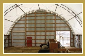
The end-wall of this hoop building has been totally framed up and skinned with metal. The framing allows for easy installation of various door configurations. Note the heavy duty tubular trusses, cable cross bracing and tubular purlins (pipes running between the trusses).
