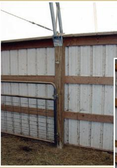
Above: The arched trusses of the Post building are bolted to the top of 6' x 6' treated wooden posts, which are set in concrete about four feet in the ground.
